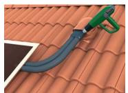
4. Shrink the shrinking tube with warm-air heater. Cable sealing is not shrunk or heated.
